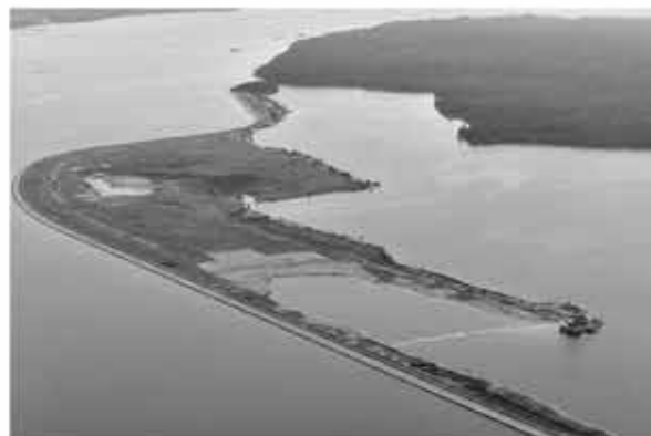
Palau Tekong under Construction
