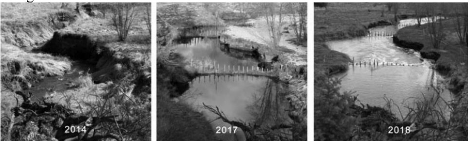
Before and after installing a Beaver Dam Analogue, Biohabitats, 2018.
