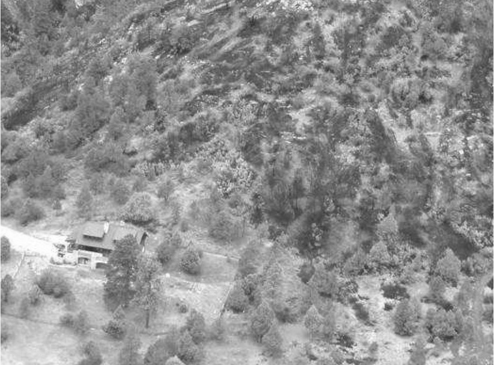
A house survived the Weber Fire near Mancos in 2012 thanks to careful planning and maintenance of defensible space, Published in the Durango Herald, 2018.
